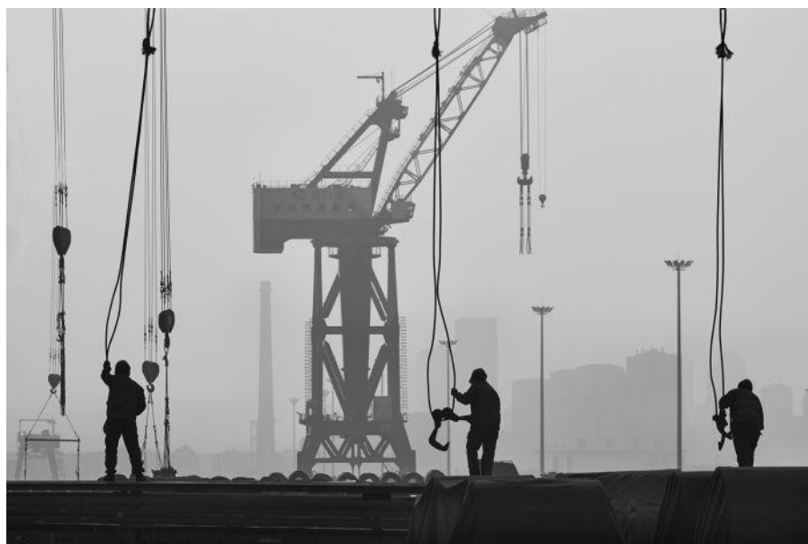
SALON HM - Yi Wu, China, Construction Site
