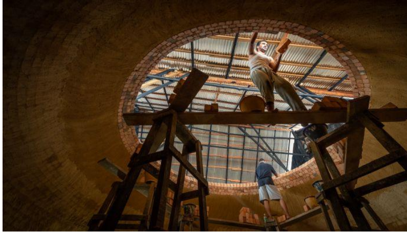
SALON HM - JIN HUAT YEOH, Malaysia, Bricks to build Charcoal Kiln
