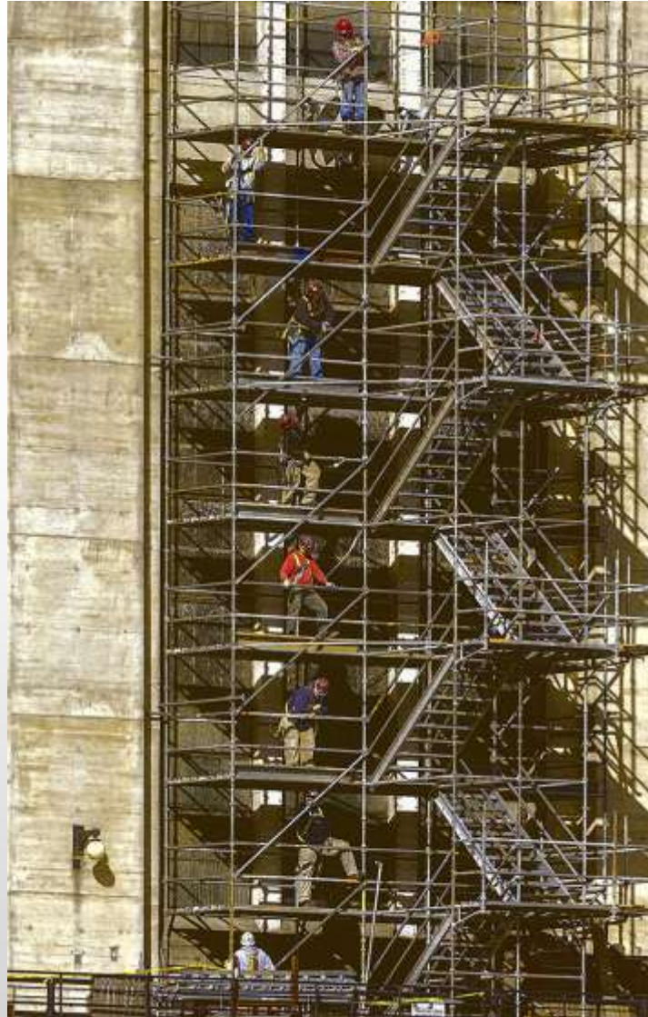
SALON HM - Hung Ta, USA, construction
